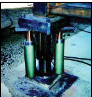
Contractors called on the brute force of Simplex R5513 cylinders to lift and position highway ramps in San Diego. G6 provided the power and control in this rough outdoor application.
